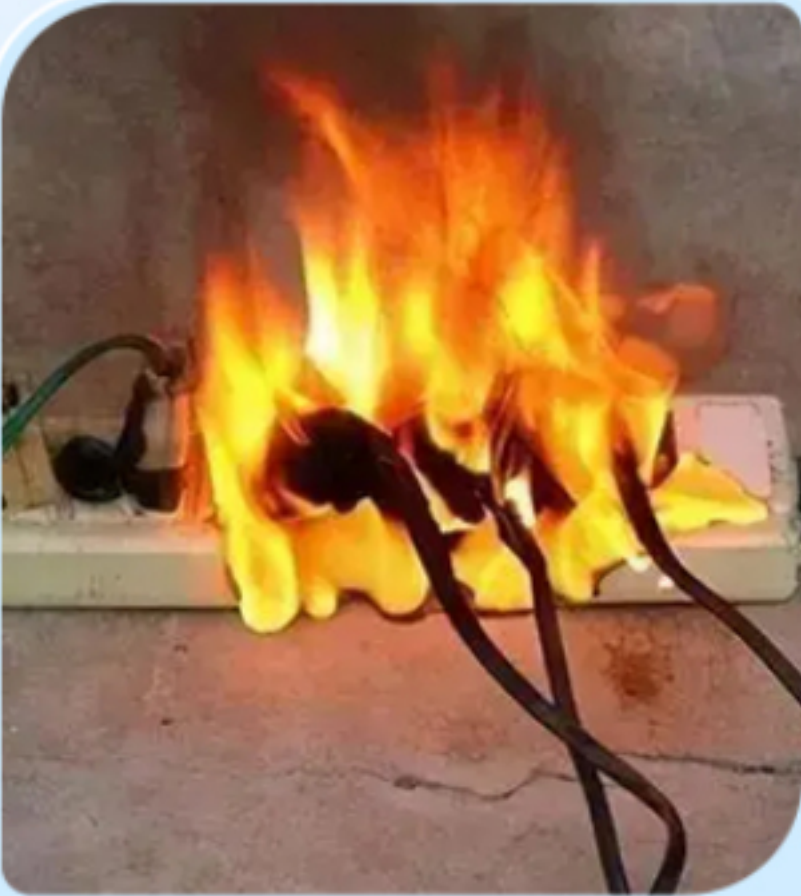
Electrical Appliances Overloaded, Causing Socket Fires
