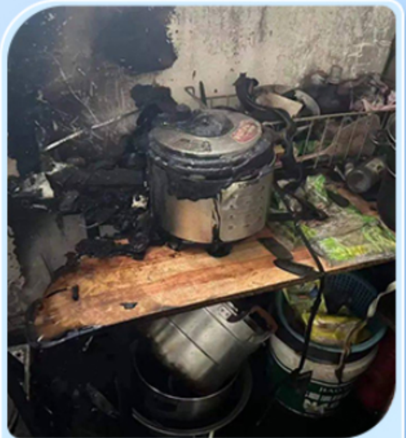
In damp zones like kitchens and bathrooms, wet inner wires spark disaster.
