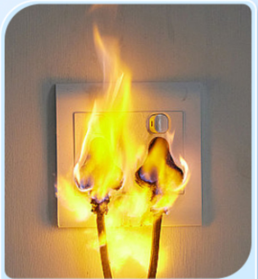
Socket Surfaces Overheating, Power Strip Plugs Discoloring
