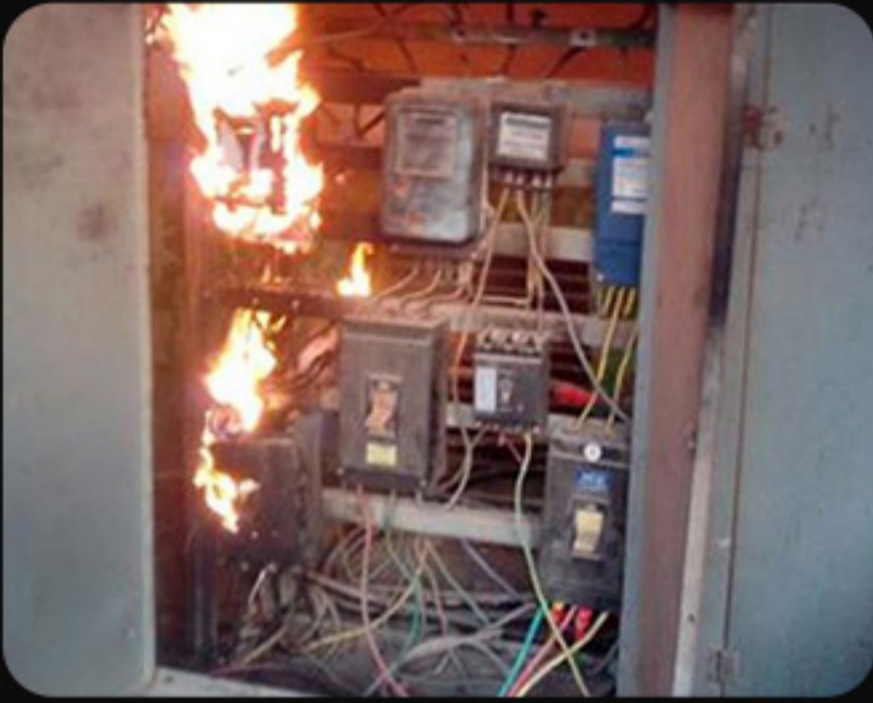
Aging electrical circuits
