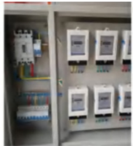
Electricity meter boxes
